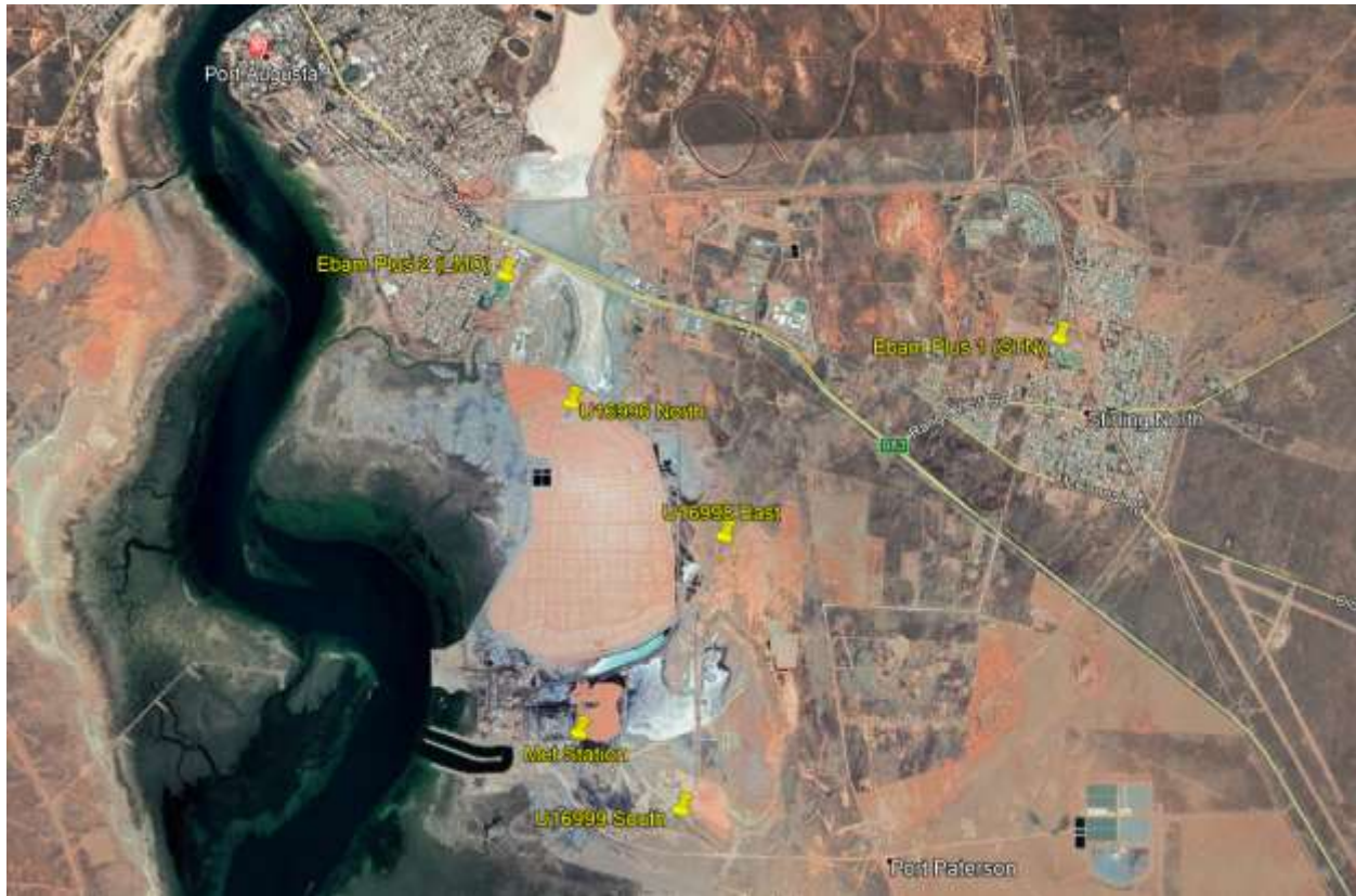
Figure 1: Port Augusta Operations Monitoring Stations Locations
