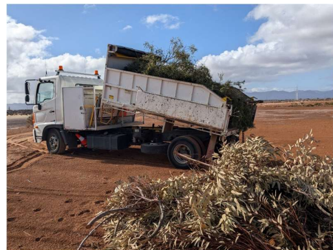
Council organic material delivered to site
