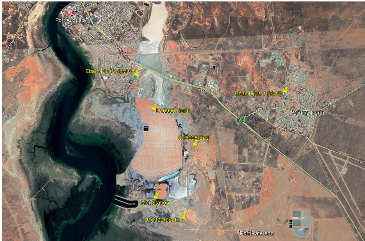
Figure 1: Port Augusta Operations Monitoring Station Locations
